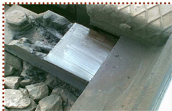
Railroad switch lubrication
